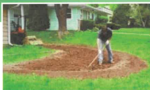
On a gentle slope, soil from digging out the garden can be used to create the berm.
